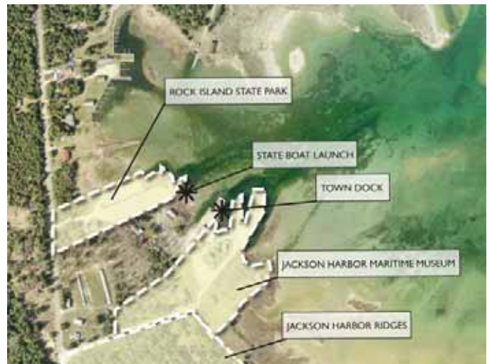
Aerial view of Jackson Harbor facilities
