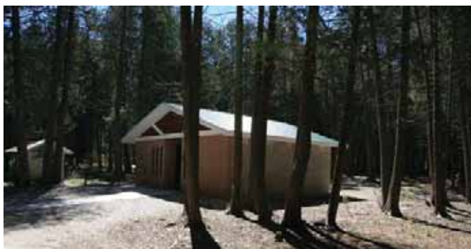
New restroom facilities are nestled into the landscape
