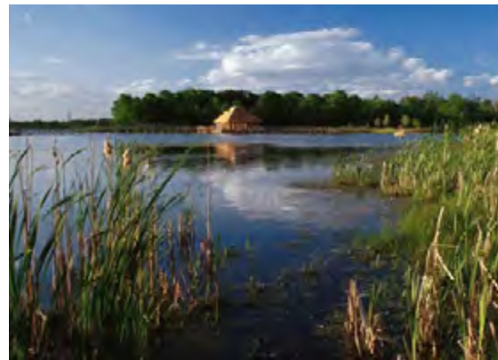
Shelter built into pier (Crosswinds Marsh, MI)
