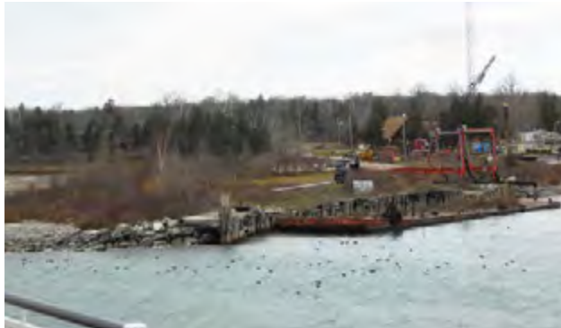
Existing view of Kap's Marina as approaching the harbor
