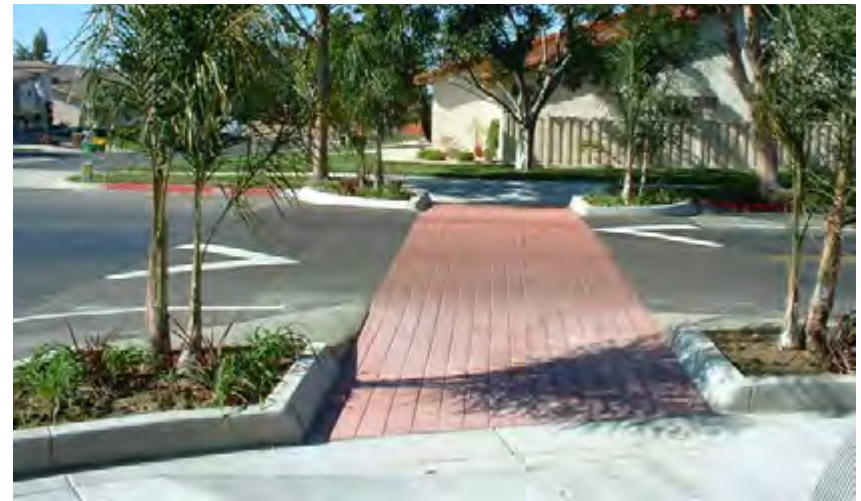
Raised crosswalk with bulb-outs (Florida)
