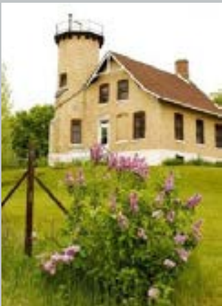
Chambers Island Lighthouse (Source: Town of Gibraltar)
