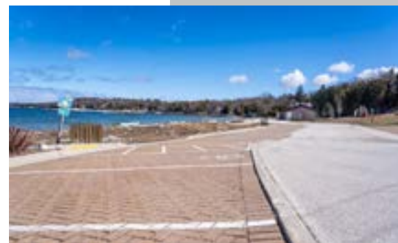
Porous pavement and natural berm in the Village of Egg Harbor to prevent runoff and decrease water contamination, Rachel Lukas, Door County Pulse
