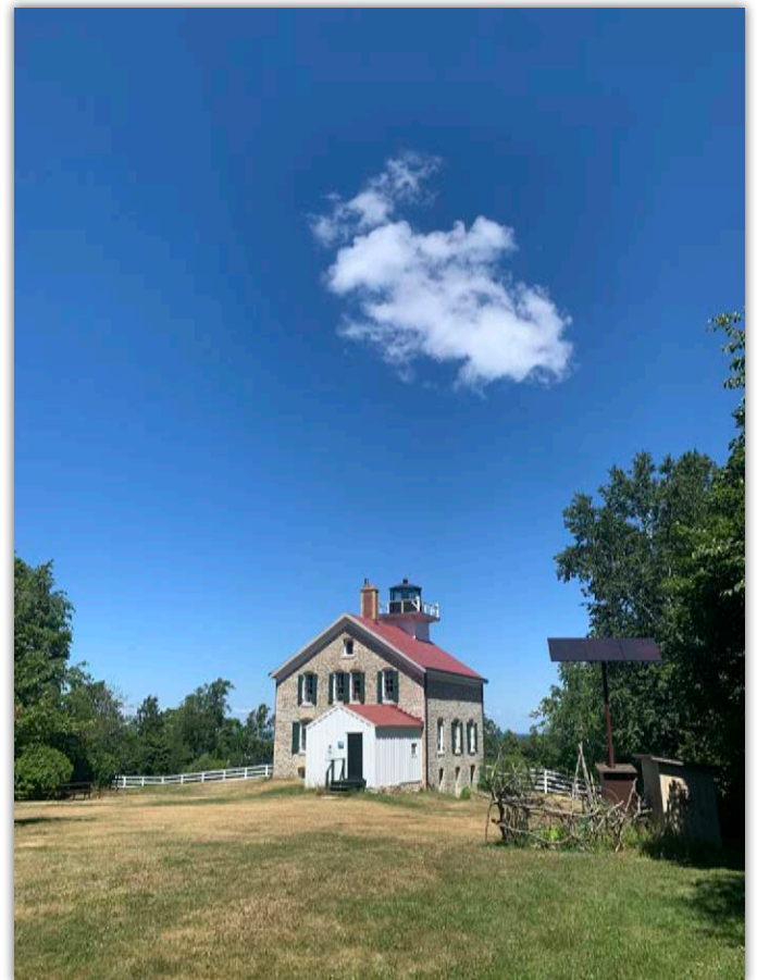
Pottawatomie Lighthouse on Rock Island State Park
